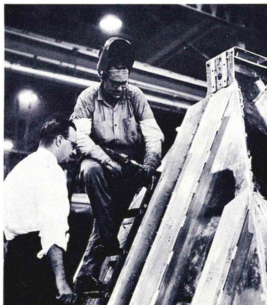
Vasin checks with Elva Ratliff, and keeps close tabs on the welding operations.
